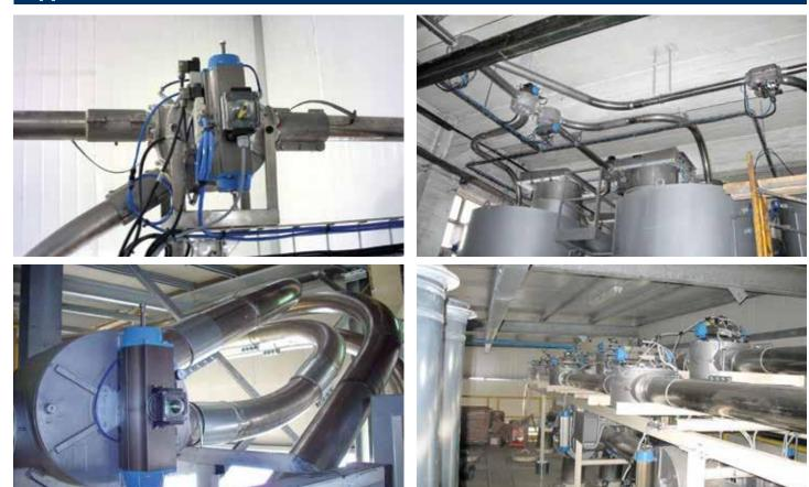
VAR Drum-Type Diverter Valves are essential components of all kinds of pneumatic conveying systems in those points where the material flow has to be diverted from one duct to another.
